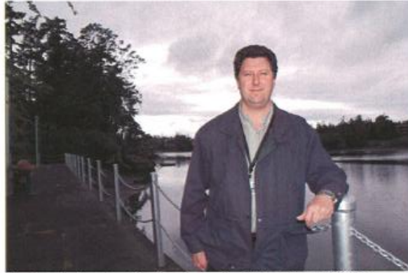
Esquimalt's director of engineering and public works, Jeff Miller, stands at the Arm Street seawall that is slated for repairs this summer. Erin Cardone/News staff
